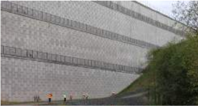
45 meter high tiered wall - SeaTac airport - USA
